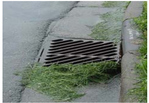
Grass clippings can clog drainage pipes and can cause algae blooms and fish kills in our creeks.
